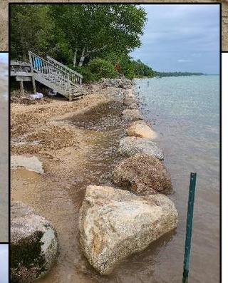
Above, end August. Breakwater as built. Stake marks OHWM 20 inches down **Water level 582.2**
